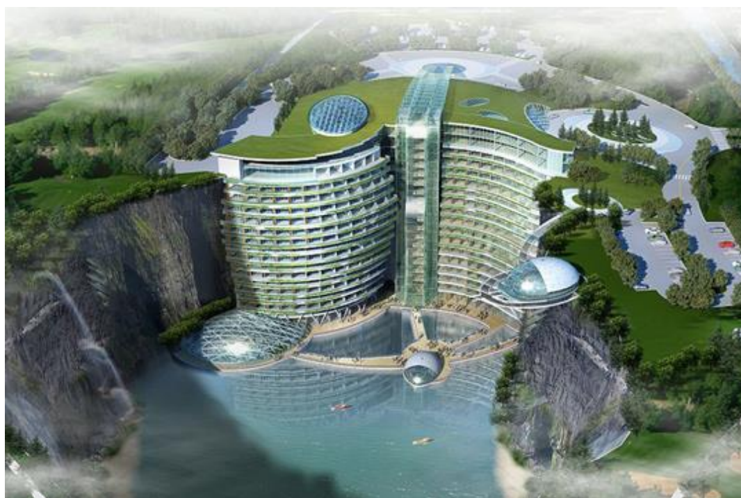
Rys. 12. Hotel – Kompleks Shimao Wonderland Intercontinental (fot. Atkins)
