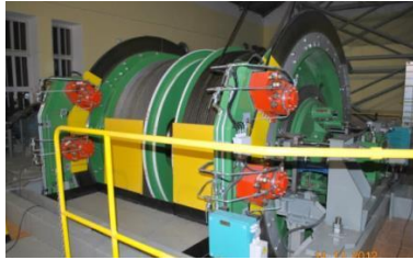
Fig. 1. Double-drum hoisting machine Kinga Shaft
