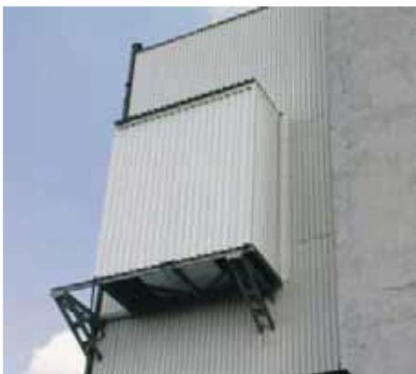
**Fig. 18.** Silencer of the air draw and ejector installed at the Jankowice Mine [17]
