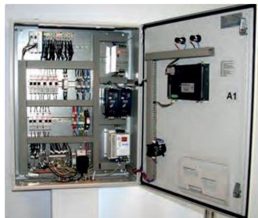
**Fig. 21.** Control system of the laboratory test rig
