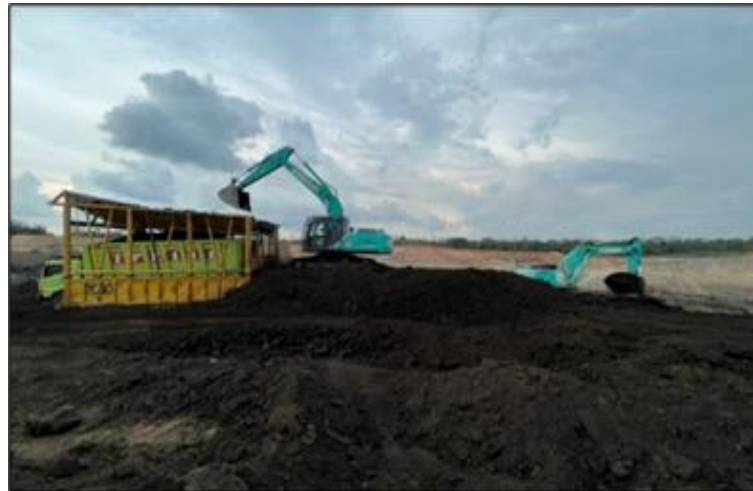
Fig. 4. Coal Extraction with In-pit Processing
