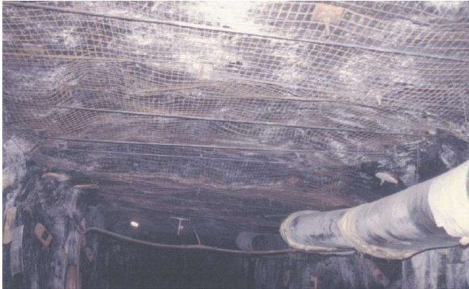
Fig. 3.19. Bolting-strand support with steel ropes in the heading working [104]
