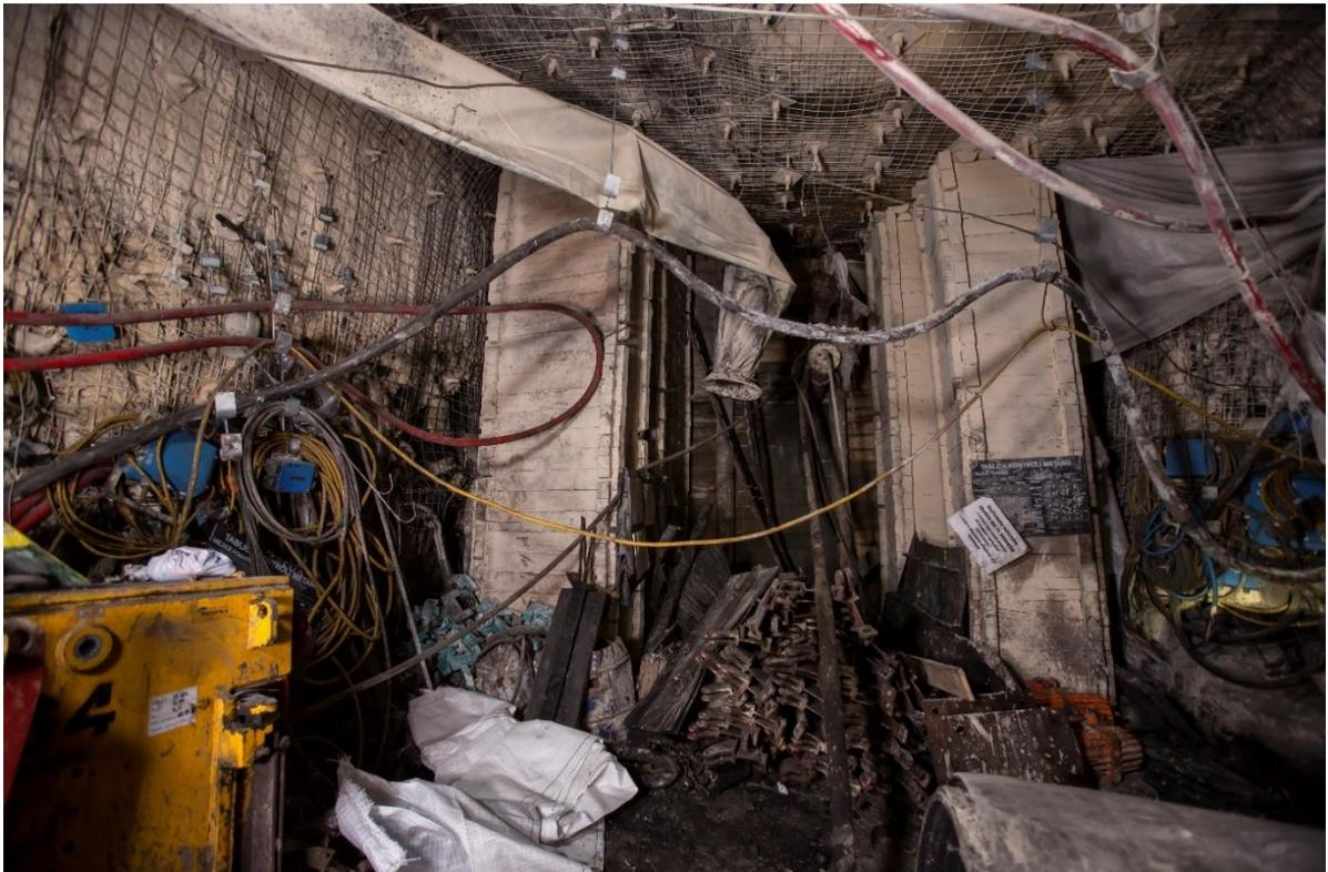
**A view of cribbing in the area of Bw-1n roadway bend in Budryk coal mine**
