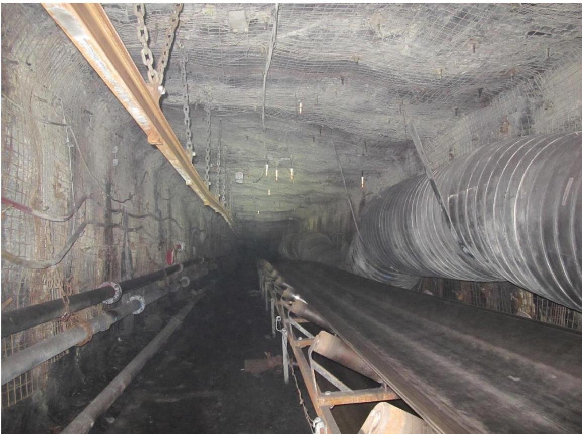
**A view of the initial section of Bw-1n roadway supported with independent rock bolting in Budryk coal mine**
