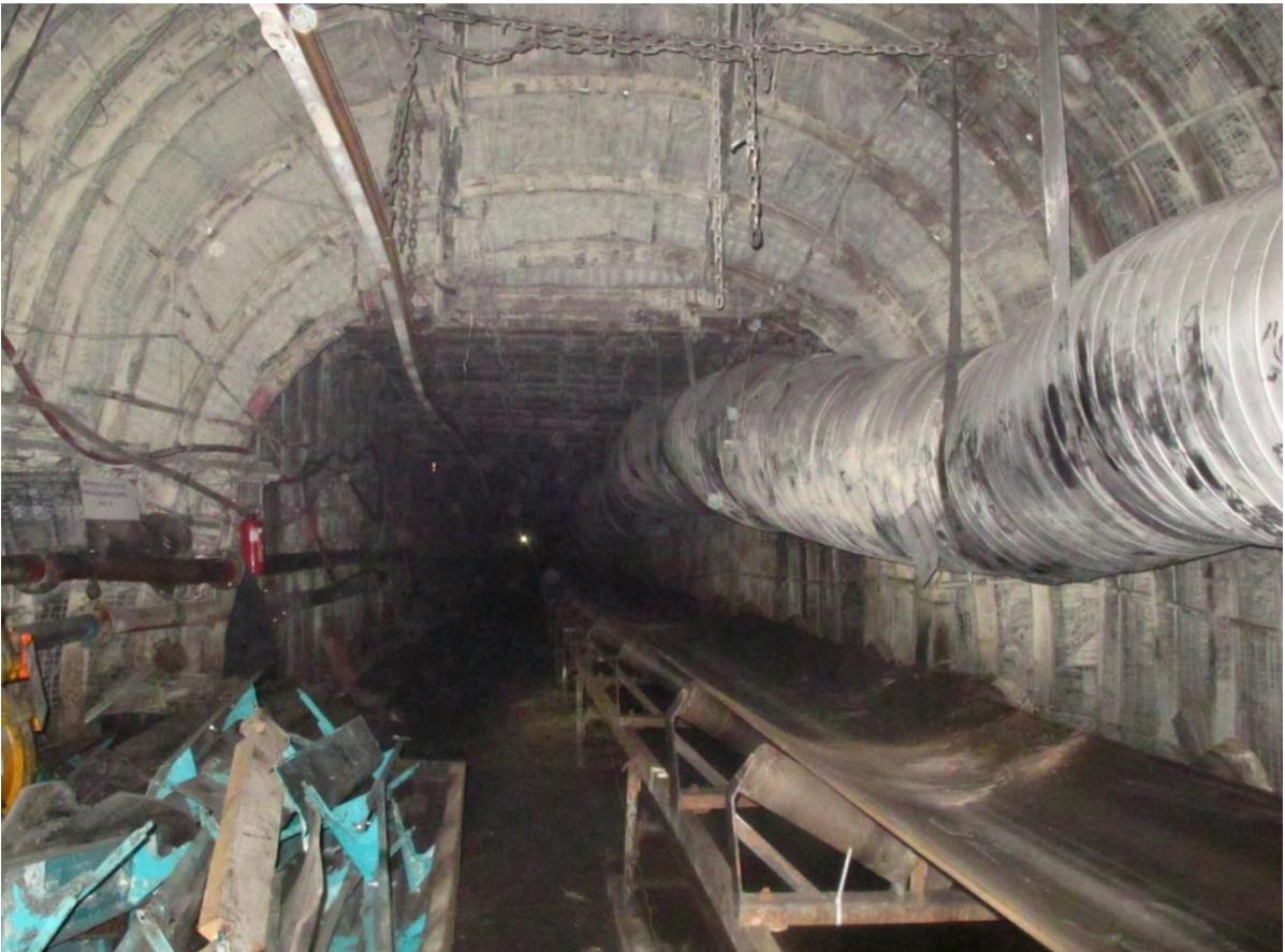
**A view of the initial section of Bw-1n roadway supported with steel arches in Budryk coal mine**
