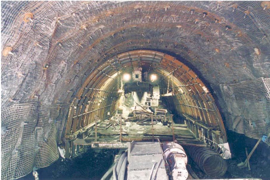
Fig. 3.9. A view of gateroad driven in the mixed support of type A [64]
