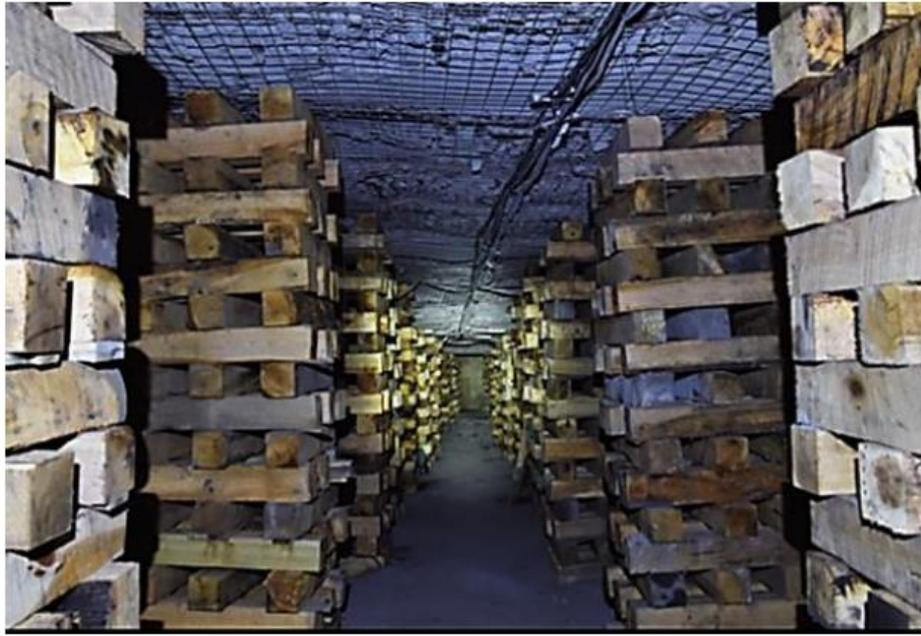
Fig. 3.11. Roadway driven in independent bolting support strengthened with wooden chocks [85]
