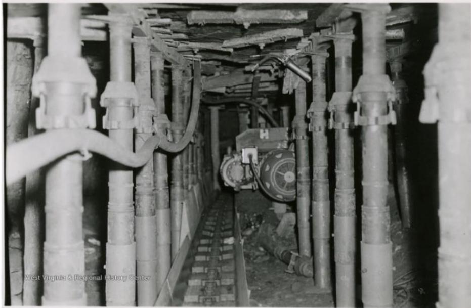
Fig. 2.1. Tailgate with a scraper conveyor and additional enforcement with steel props in the longwall area [4]
