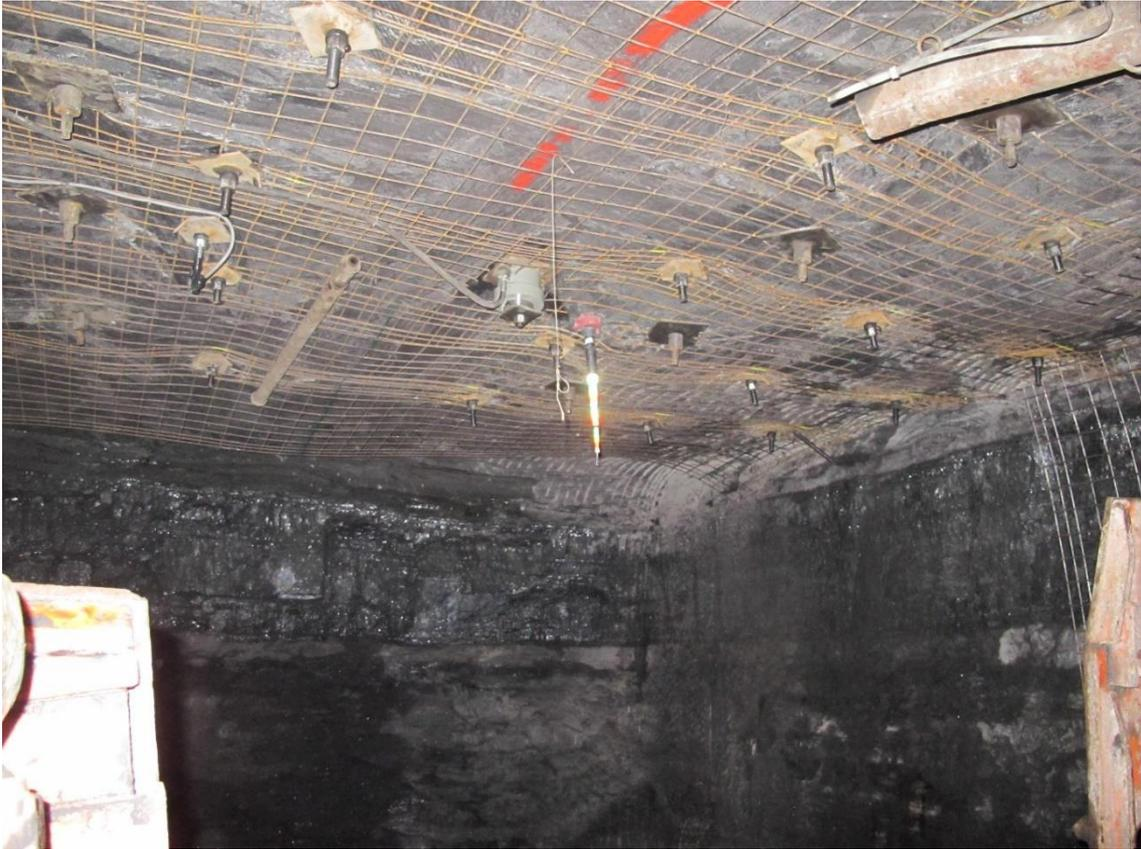
**A view of an extensometer installed in the roof of Bw-1n roadway in Budryk coal mine**
