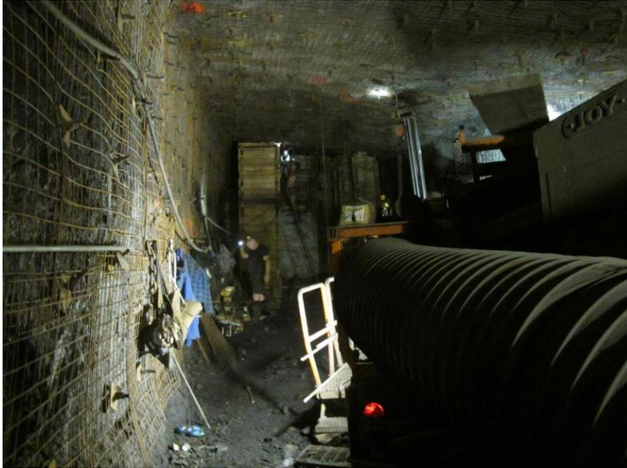
Fig. 11.18. Driving the bend No. 2 - chocks [132]
