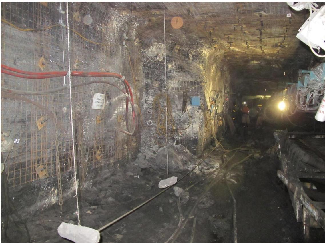
**Widening of Bw-1n roadway supported with independent rock bolting support in Budryk coal mine**
