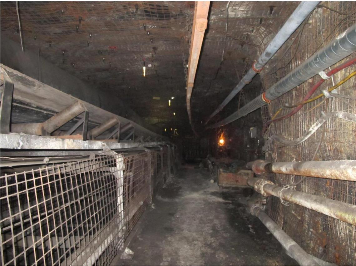
**A view of Bw-1n roadway supported with independent rock bolting in Budryk coal mine**
