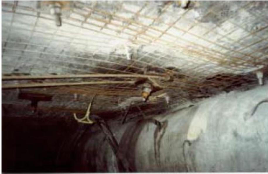
Fig. 3.18. Bolting-strand support with steel ropes before applying initial tension [95]
